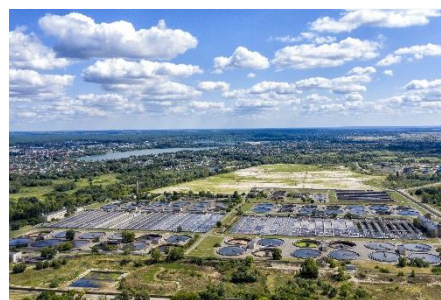
Wastewater Treatment Plants (WWTP)
