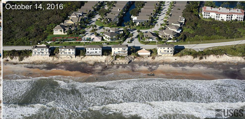
Vilano Beach after Hurricane Matthew
