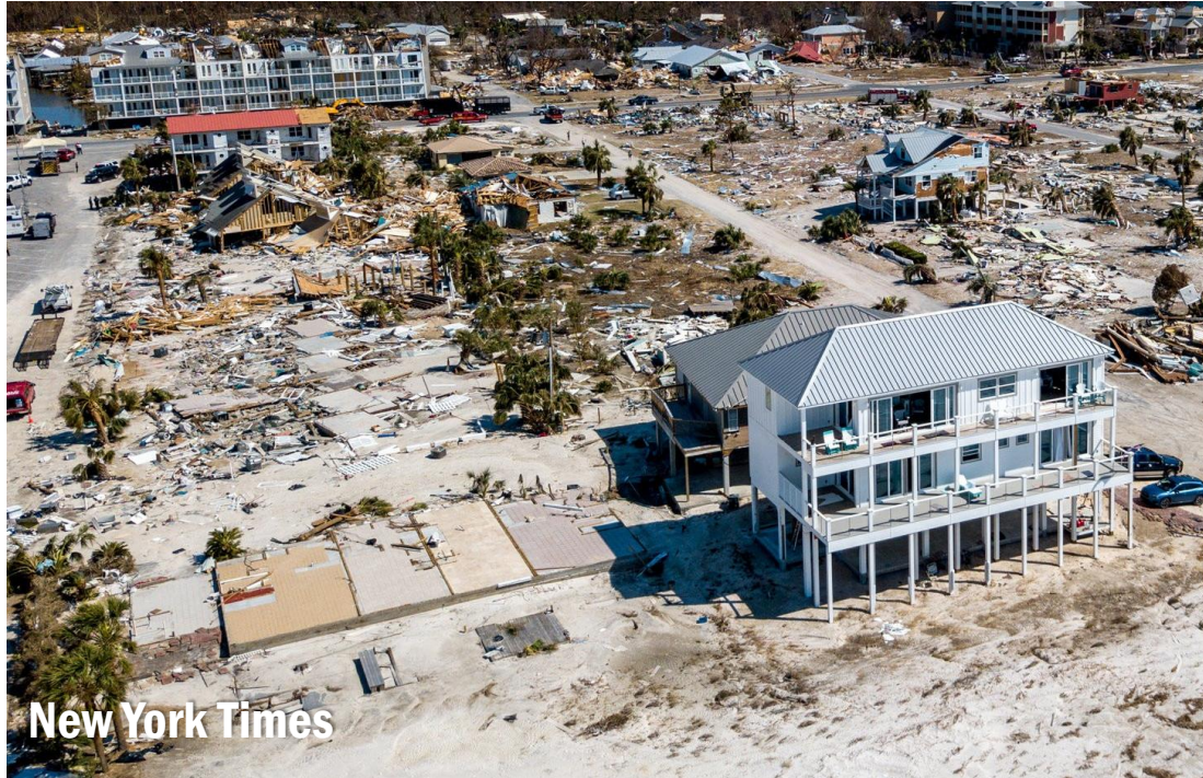
Mexico Beach after Hurricane Michael
